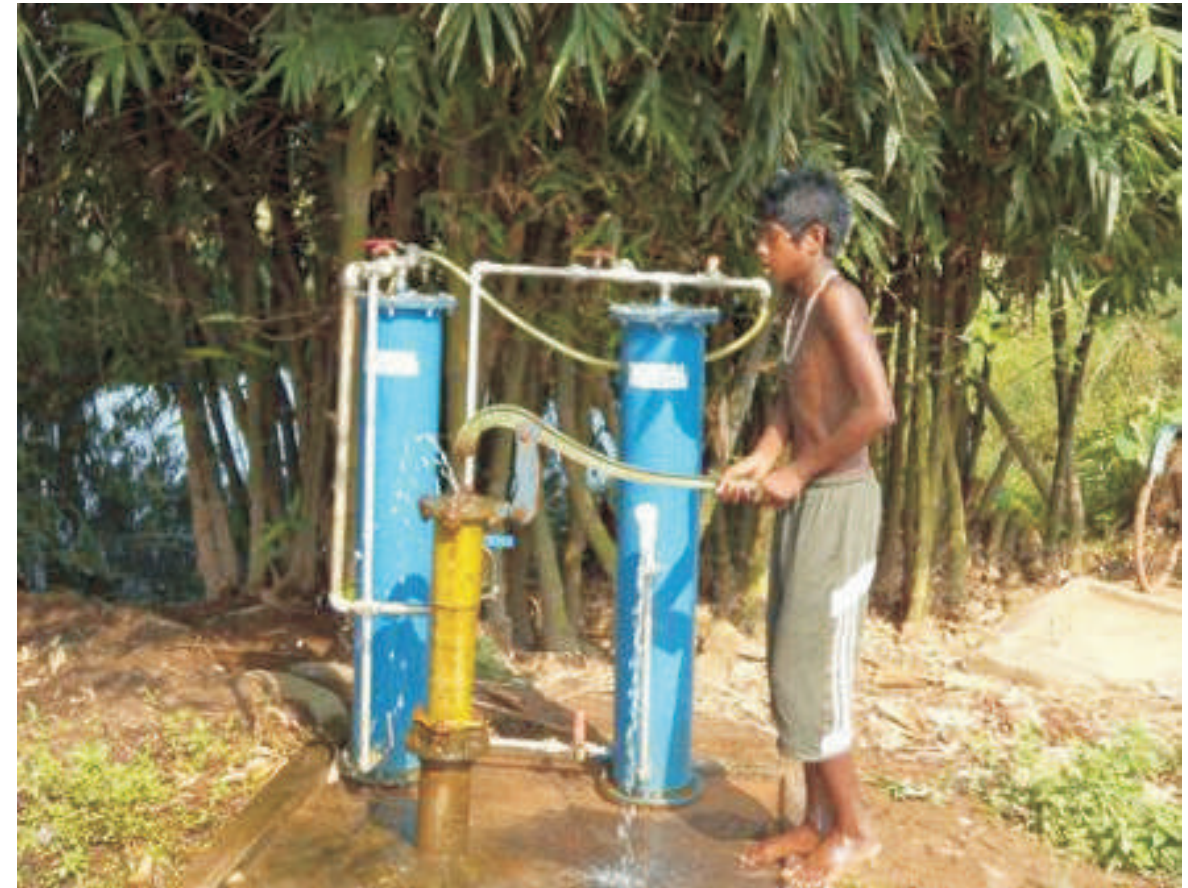
(Photo of the Govt. recommended treatment method at community level being used in Bihar to be shared)
